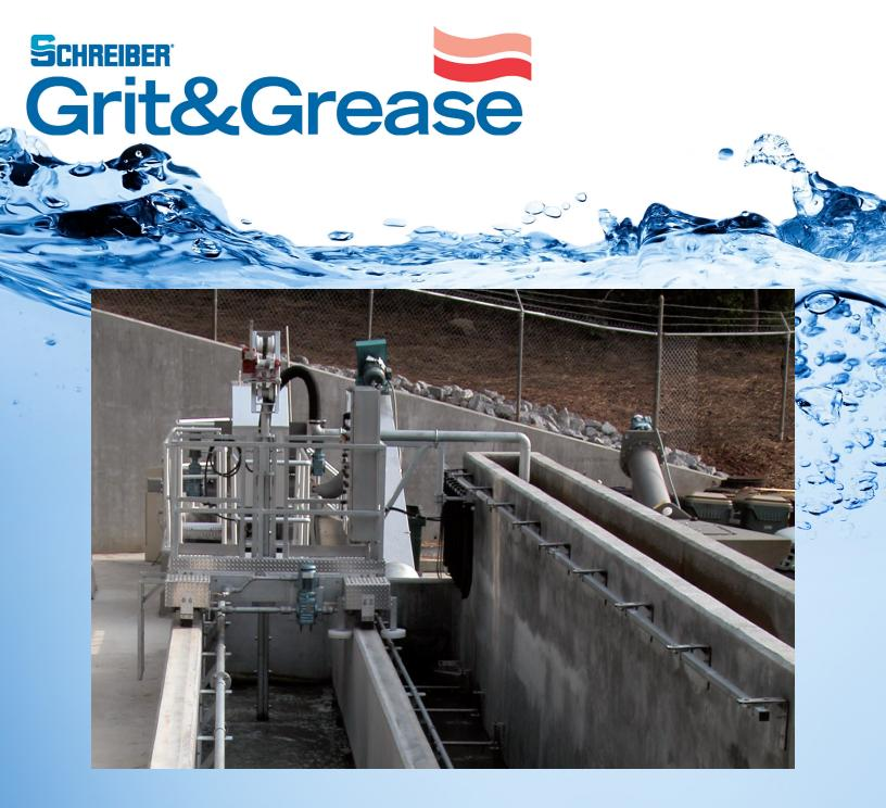
Schreiber's Grit & Grease removal system is a unique system designed to remove both Grit and Grease in a common structure.
